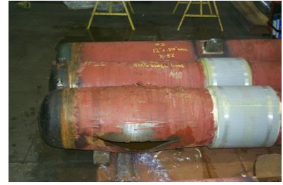
Pipe Body Failure @ 4,260 psi
