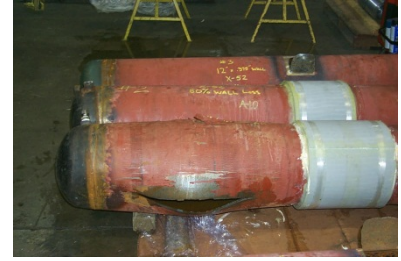
Pipe Body Failure @ 4,260 psi
